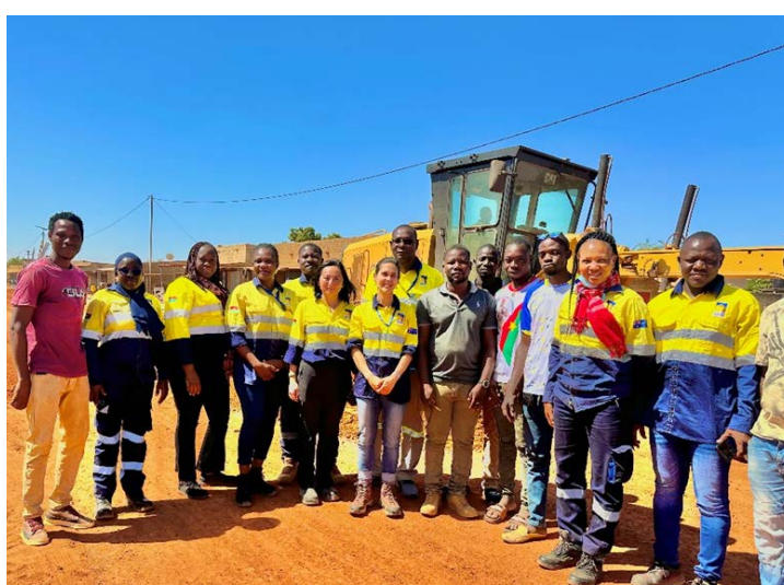
Rehabilitation de la route
